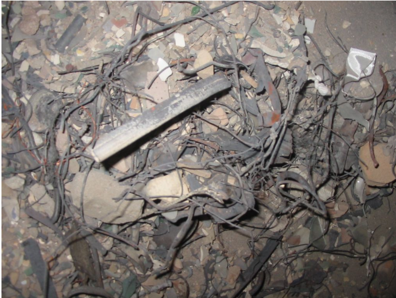
Bed Plugged with Wires and Coarse Material
