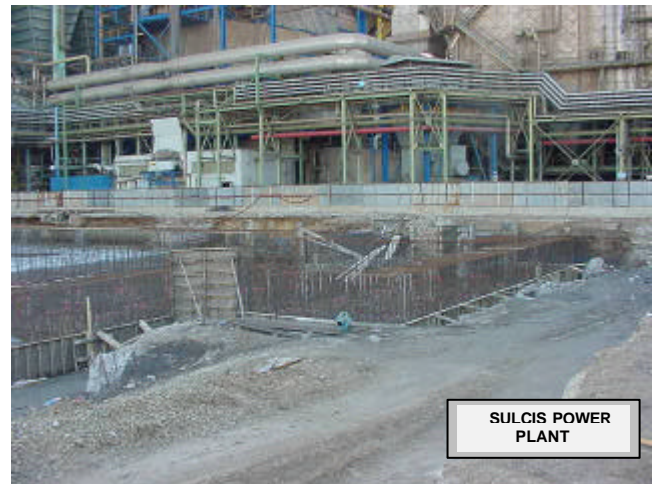
Figure 7 Working to Boiler Foundation in progress at the beginning of 2002
