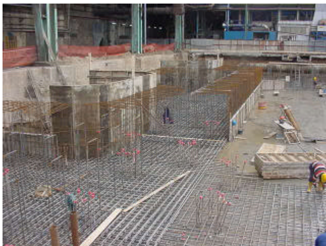
Figure 6 Working to Boiler Foundation in progress at the beginning of 2002
