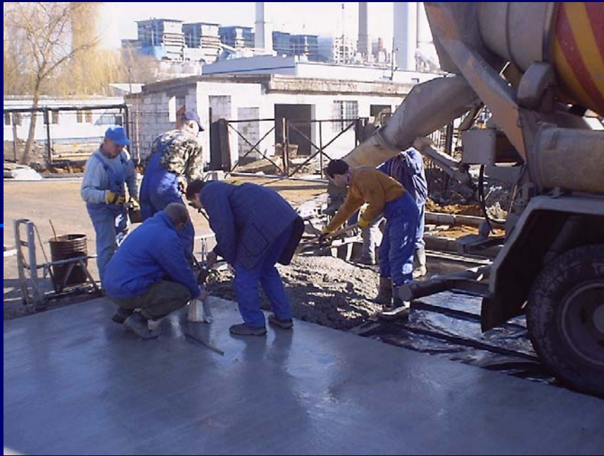
Test section of the road at power station in Turów
