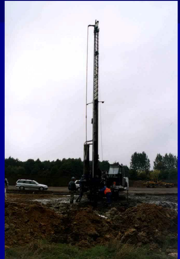
Ground strengthening by injection – highway A4
