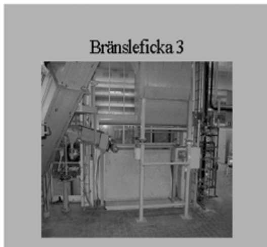
The third fuel hopper for dry sludge and other secondary fuels
