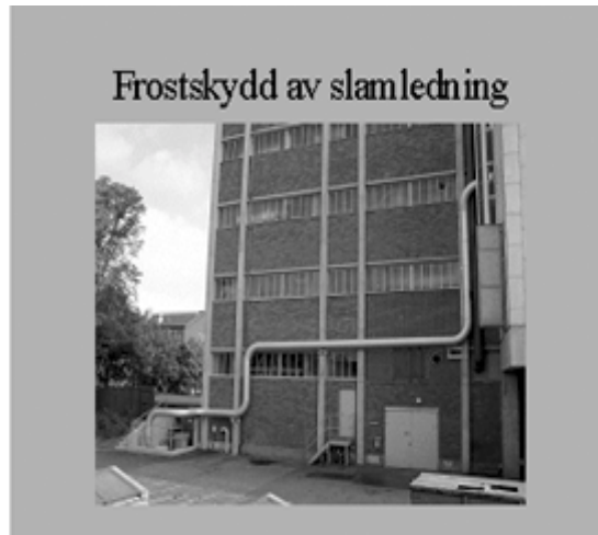
Freeze protected duct for sludge feed to the boiler.
