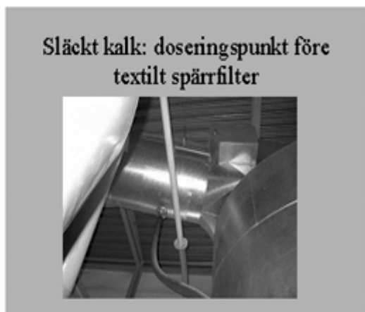
Feed point for calcium hydroxide upstream of the bag filter.
