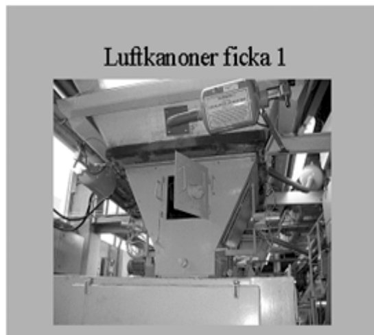
Air blasters for the two main hoppers originally built for coal.
